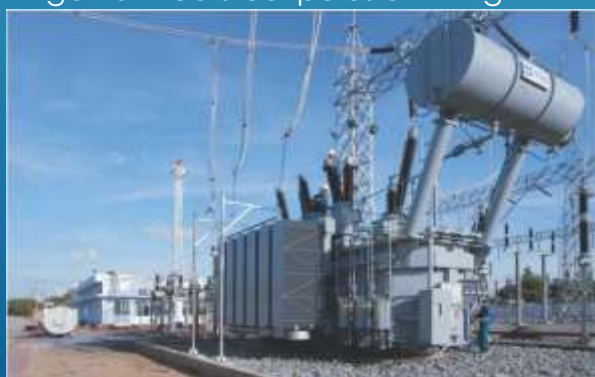
Lắp đặt tủ & panel Trạm biến áp 220 kV - Tiền Giang / Installation of cabinet & panel for 220kV Transformer Station – Tien Giang
