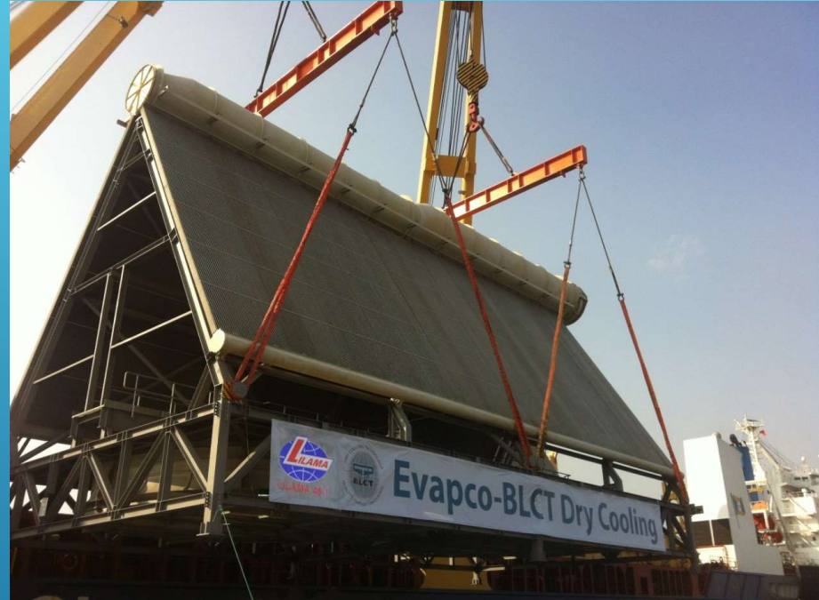
Loading out the Module ACC for Ichthys Onshore LNG Facilities Project
