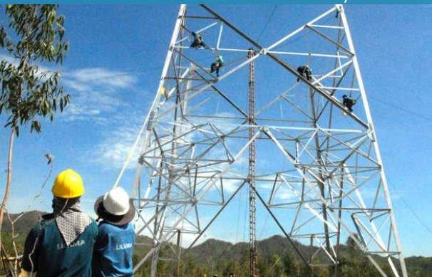
Lắp đặt đường dây 500 KV Vĩnh Tân – Sông Mỹ / Installation of transmission line for Transmission line 500kV Vinh Tan - Song May
