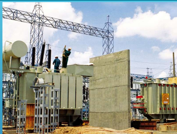
Lắp đặt 01 MBA 125 MVA, 05 nhánh 220KV, 07 nhánh 110KV/ Installation of 01 Transformers 125 MVA, including 05 Route 220 KV and 07 Route 110 KV
