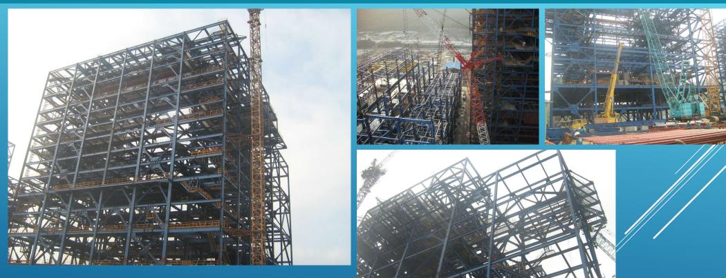
Installation of steel structure for Vung Ang 1 Thermal Power Plant
