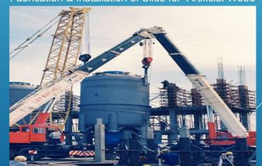
Installation of Steel structure, Equipment, piping for PVC plant
