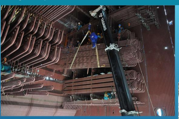
Installation of 1,180 tons Boiler for O Mon 1-2 Thermal power plant
