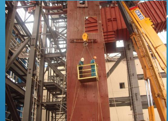
Installation of Boiler drum, Furnace water wall for O Mon Thermal Power Plant Unit No.1
