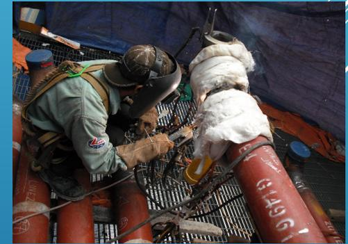
Installation of SH spay, SSH outlet, RH outlet for Vung Ang 1 Thermal power plant
