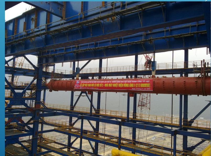
Installation of Boiler drum 311 Ton for Vung Ang 1
