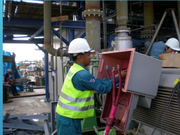
Connecting of medium voltage cable 6.6KV to switchboard
